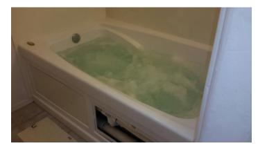
12.12 - The hydro-spa does not appear to have ground fault protection, which is an essential safety feature that should be be verified as being present or added.
