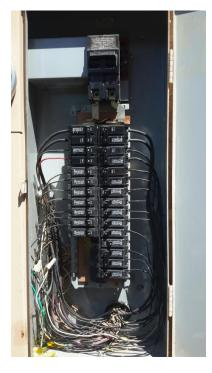
6.10 - There is modern aluminum wiring in the panel but only on the larger circuits such as: the range and a/c unit.
