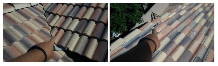
9.4 - Viewed at least 10 out of place roof tiles that should be evaluated and repaired or replaced as necessary by a qualified roofer or technician. These issues should be repaired to help prevent wearing of the protective layer beneath the roof covering or possible moisture intrusion within the residence. They were located at the very top middle north side.
