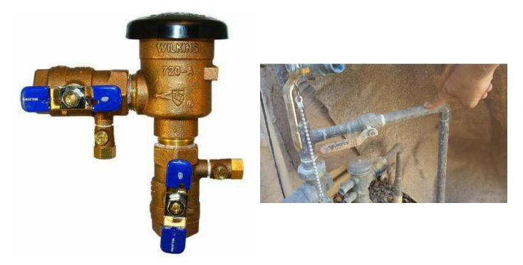
16.11 - The backwash valve in the pool equipment area leaks allowing water to pass through it, which should be serviced as necessary by a qualified pool technician.
