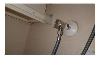
12.10 - In the master bathroom there are calcium deposits or build up on the drain line that could indicate a slow or previous leak. However, this area was not wet or leaking during the inspection. Right sink
