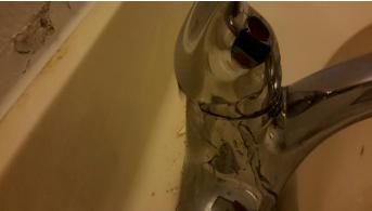
11.8 - In the master bathroom corrosion and/or mineral build-up was observed on the master bathroom Right and left shut-off valve. This corrosion or build-up may prevent the shut-off valve from working properly, especially if emergency shut-off is needed. I recommend a qualified, licensed plumber should evaluate and repair or replace this valve or connection as necessary.
