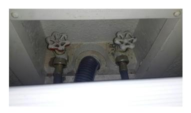
3.6 - The water supply to washing machines is commonly left on, and the rubber hoses that are commonly used to supply water can become stressed and burst. For this reason we recommend replacing all rubber supply hoses with metal-braided ones that are more resilient.
